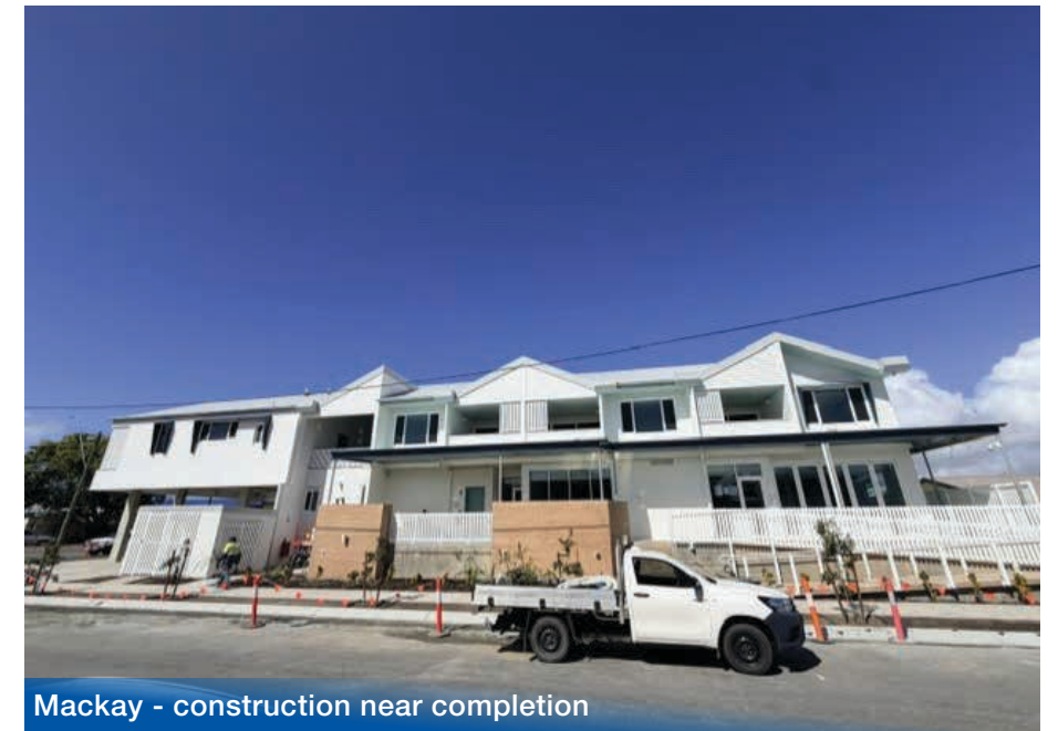
Newtown - construction near completion
