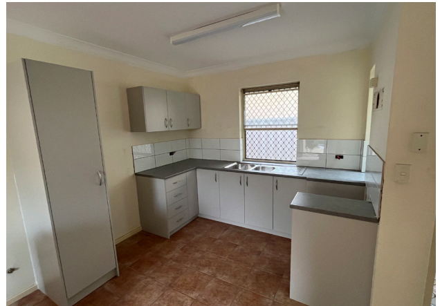
Renovations at CROFT are in full swing.
